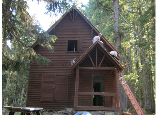
Roof reshingling at Musick Guard Station.
