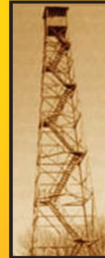
Love's Lookout City of Jacksonville, TX Love's Lookout is a remnant of a network of fire towers in the piney woods that once numbered more than 100. The 125' Aermotor tower with 7'x7' metal cab was built by the Texas Forest Service in 1935 and remained in service until 1970.
